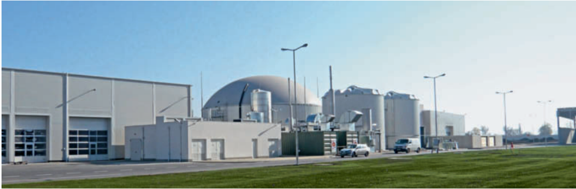
2 The combined plant for biological waste treatment in Han Bogrov was named "Building of the year – Bulgaria" in 2014
