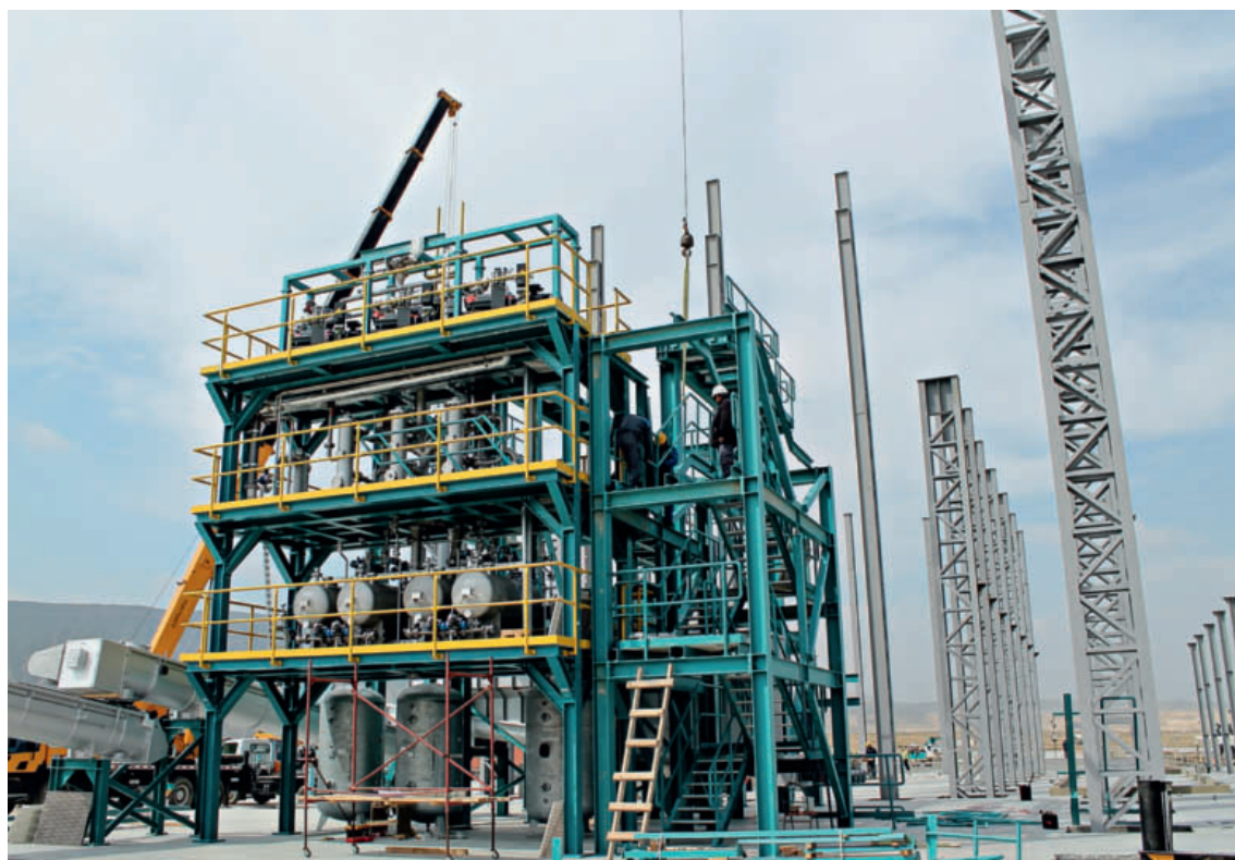
Installation of the VacuDry plant in Azerbaijan
