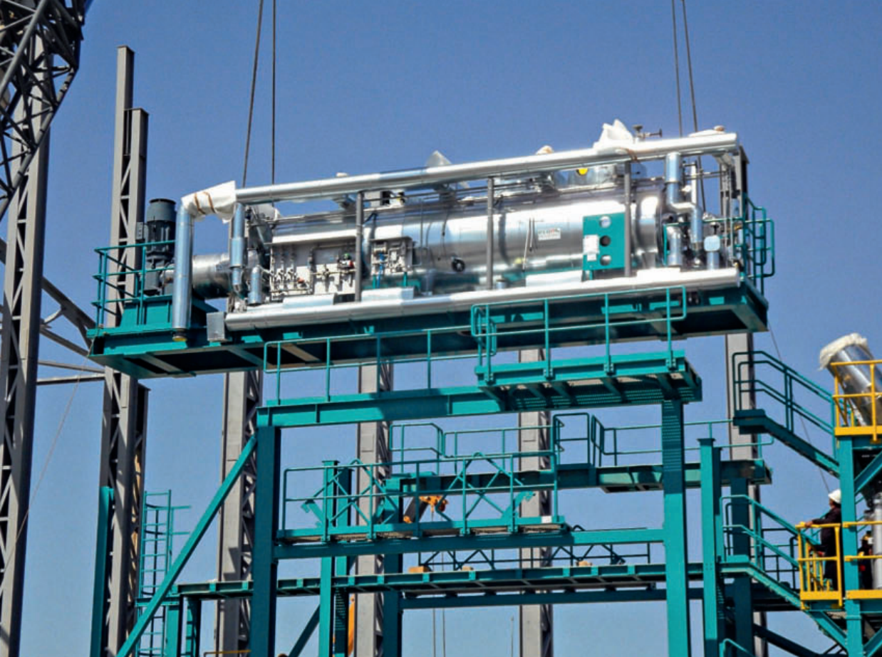
◀ Installation of the VacuDry plant in Azerbaijan
