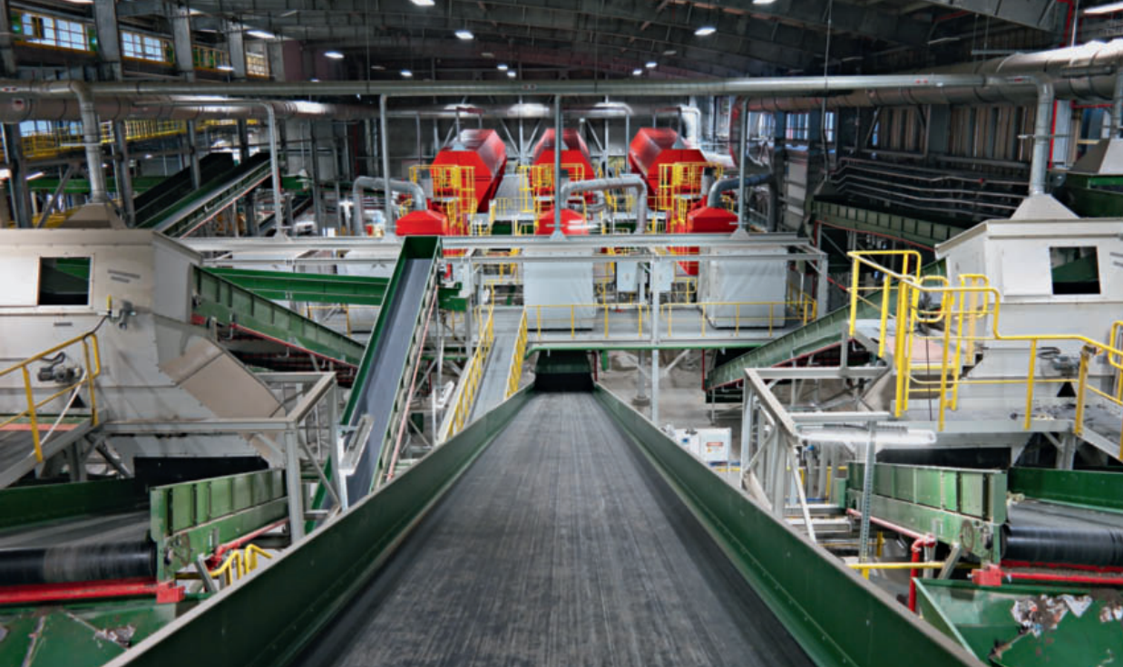
◀ RDF plant in Tel Aviv/Israel
